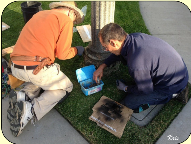
Don and Jim repair cracks in lampposts.
